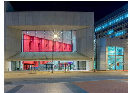
To inform administration and customers of the work that our project team was putting in place, we posted boards with project renderings showcasing the renovations.
